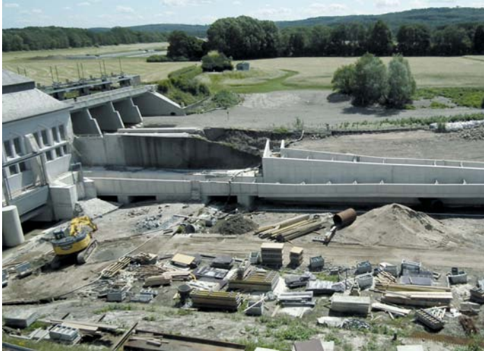
Bild 14.5: Fischaufstiegsanlage in der Bauphase Fig. 14.5: Fish migration facility during construction
