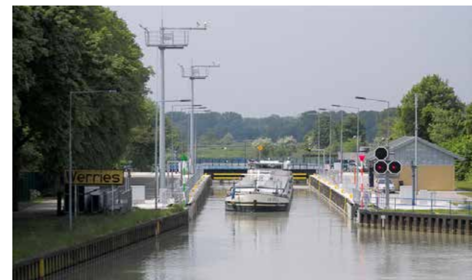
Schleuse Werries. Foto: RIK/Walter
