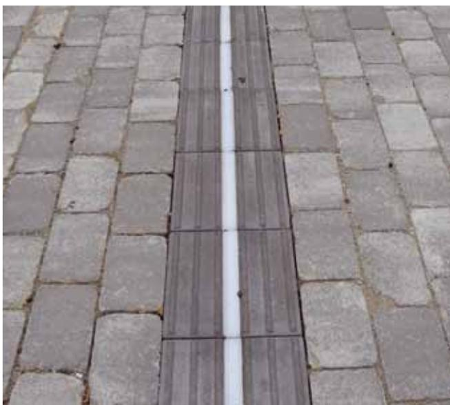
Illuminated ground surface indicator on the first test site
