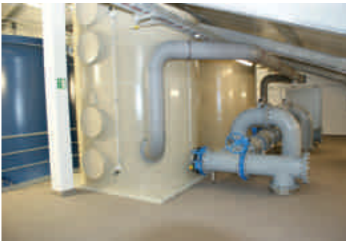
Bild 16.6: Riesler Fig. 16.6: Trickle filter
